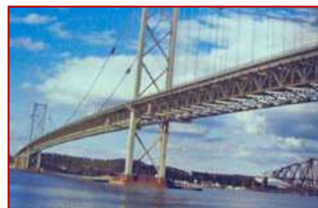
Fot. 6. Forth Road Bridge
