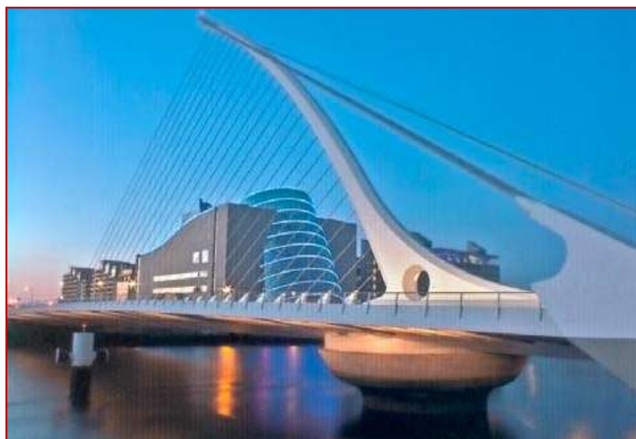
Fot. 8. Most Samuel Beckett Bridge
