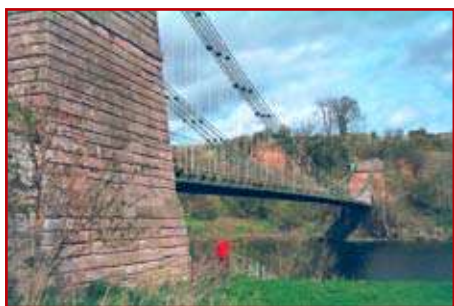
Fot. 1. Most Union Bridge
