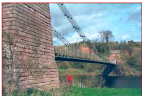
Fot. 1. Most Union Bridge
