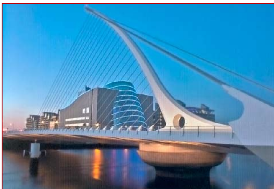
Fot. 8. Most Samuel Beckett Bridge
