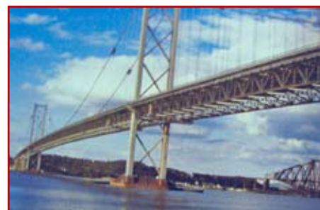
Fot. 6. Forth Road Bridge
